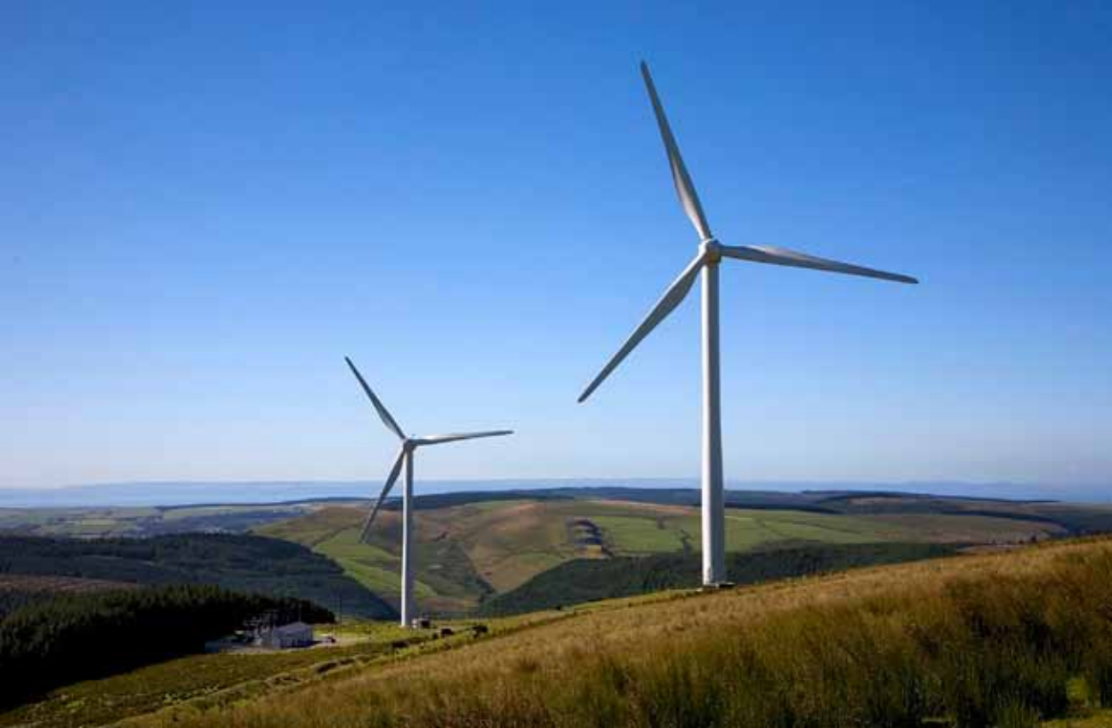
Ventient Energy's wind farm in Ffynnon Wales.
